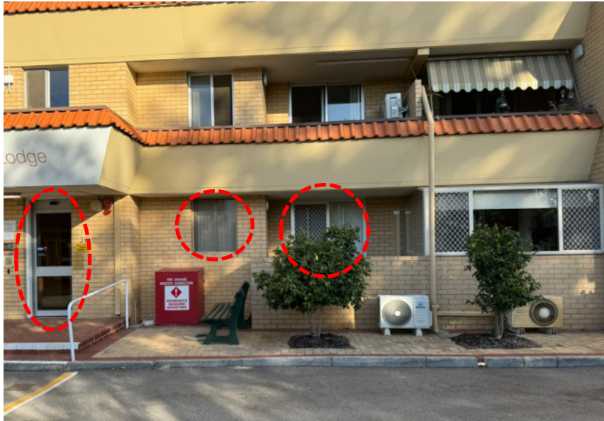
Photo 1 Openings with 2 m of Booster Cabinet
