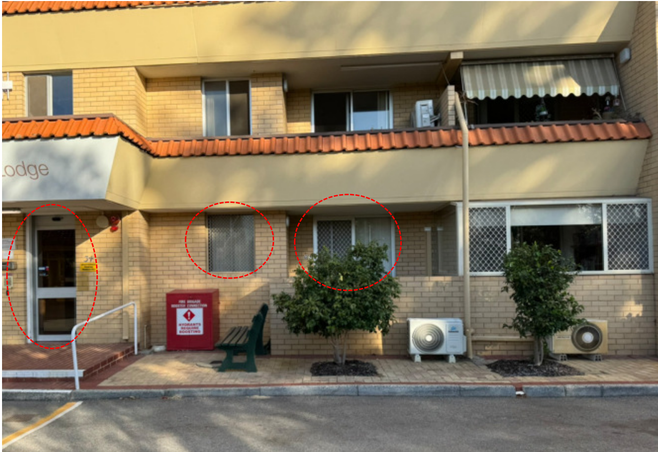
Photo 1 Openings with 2 m of Booster Cabinet
