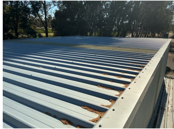
South elevation roof exterior
