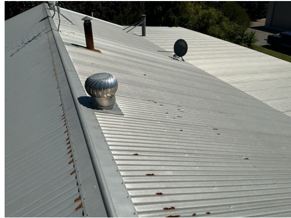
West elevation roof exterior
