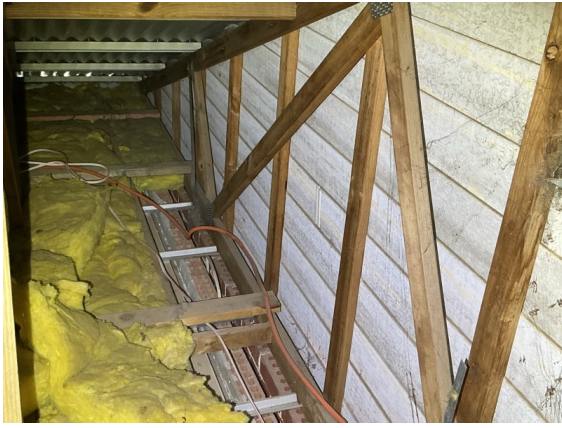
South elevation - Gable end tie down straps.
