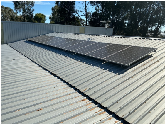
East elevation roof exterior
