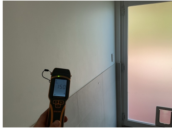
Laundry wall adjacent to the bathroom shower was checked for moisture and found to be within a normal range.
