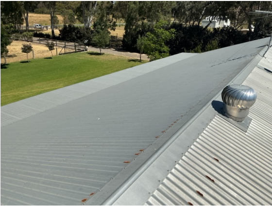
East elevation roof exterior
