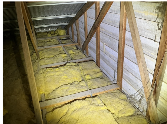
North elevation - Gable end tie down straps.
