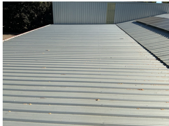
East elevation carport roof exterior
