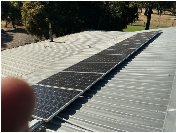
West elevation roof exterior
